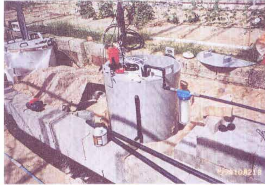
Installation of a control box
