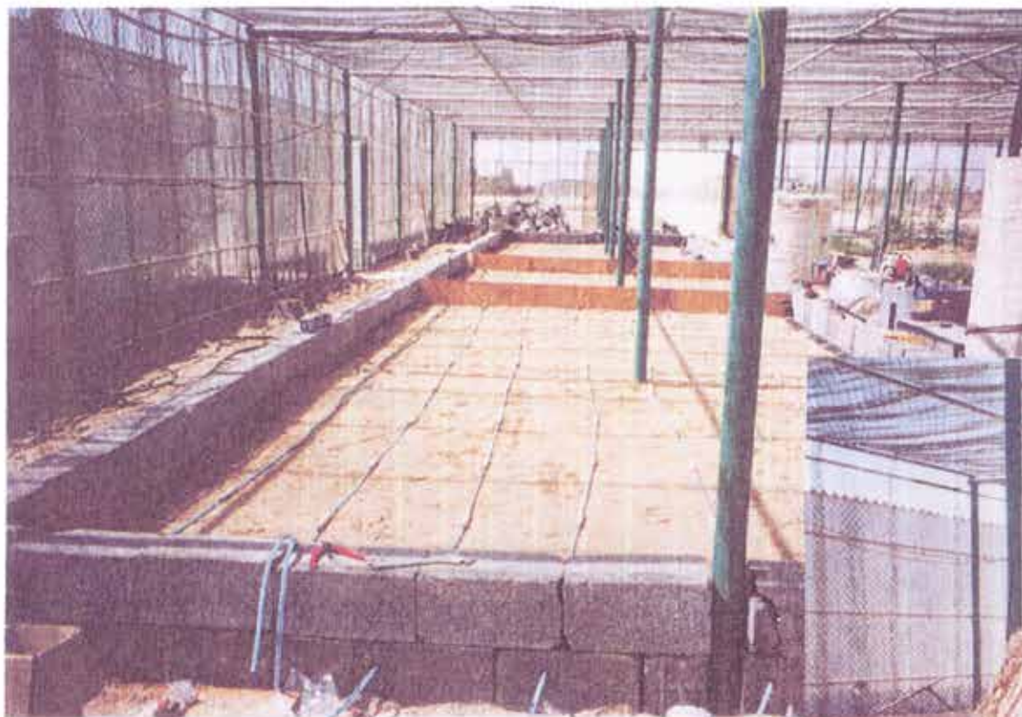
Water life system is completed
